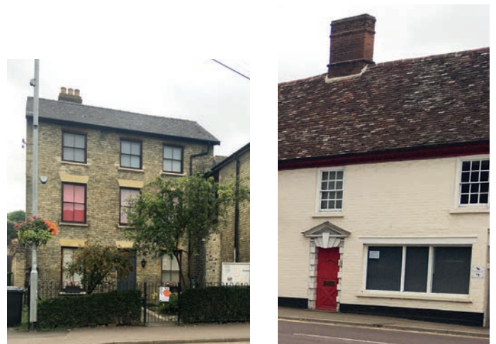
Fig 41 High Street frontages - Challis House
