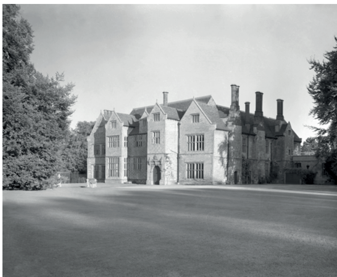
Fig 4 Sawston Hall, Grade 1 Listed Tudor Manor house
