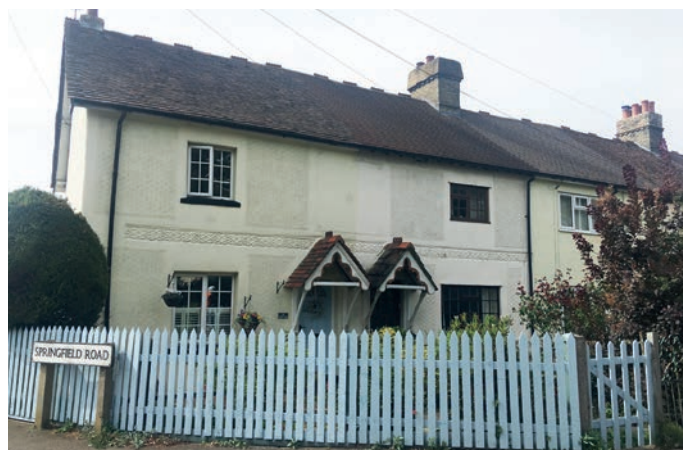
Fig 18 Springfield Road rendered terrace with decorative pargetting
