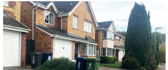
Fig 11 Detached houses with integrated garages
