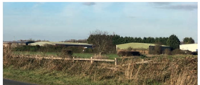
Fig 12 Large industrial units to the north east
