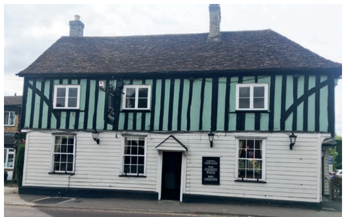
Fig 43 High Street frontages - Renovated pub
